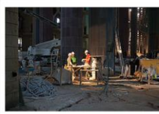
Construction workers and aerial work platforms in the nave
