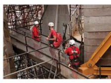
Construction workers in climbing gear on a tower
