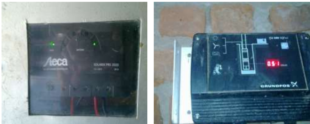
Figure 4.1:- Charge and pump controllers’ indication status for charging water pumping status at Umodzi and Kuntiyani CBOs
