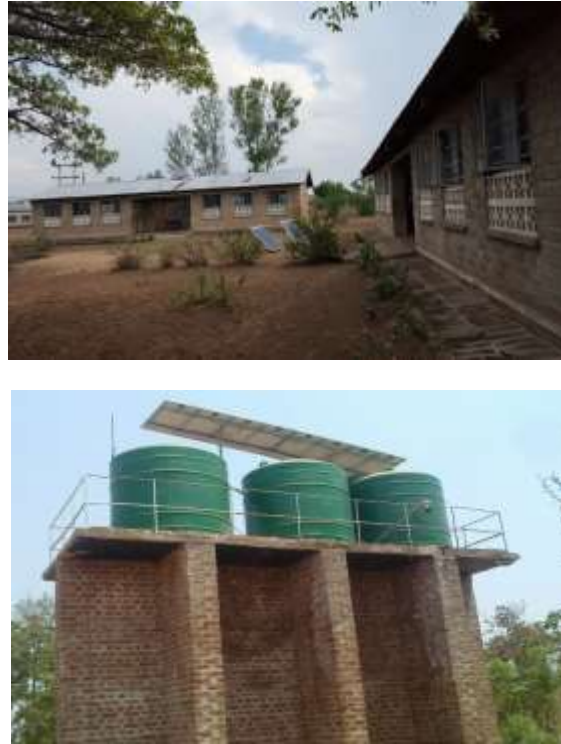
Figure 1.2:- Battery-based and water pumping solar PV systems at Umodzi and Kuntiyani CBOs.
