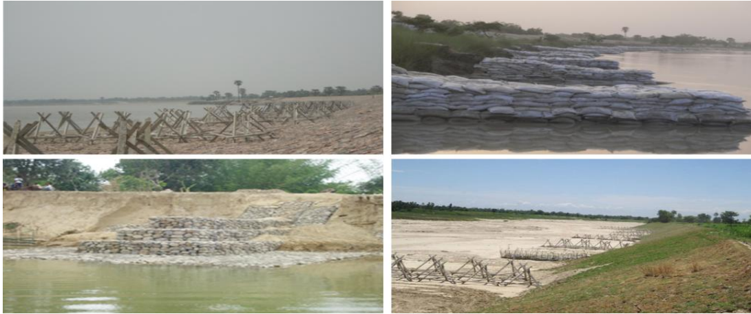
Fig 11:- Embankment and embankment protection works as structural flood control measure.
