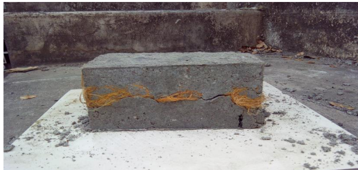
Fig.9 Failure of blocks due to the dry placement of fibers during casting
