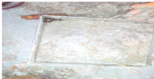
Fig.10 Application of geopolymeric slurry thoroughly to the fibers
