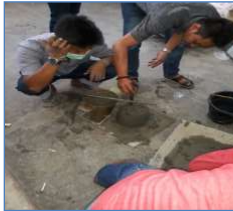
Figure 3:- Slump test process
