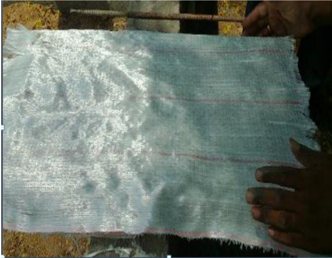
Fig 6:- Application of GFRP layer.
