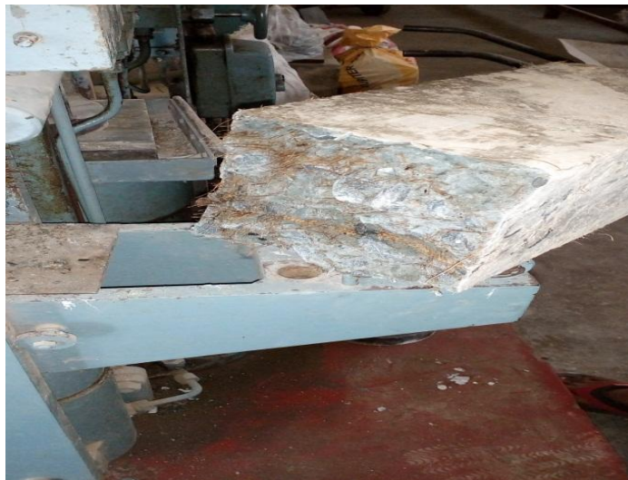
Fig 3:- C/S of beam after failure
