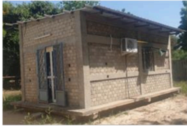
Figure 1: CABET experimental cell, seen from the north and west Representing a full-size building but of small dimensions, it consists of vertical opaque walls, two single-glazed windows, a glazed door and a roof incorporating a ceiling.
