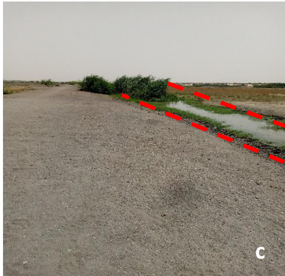
Figure 12 : Various Methods of Soil Salinity Management in Reclaimed Polders (a) Levelling with small dikes before irrigation in this wheat plot, (b) salt precipitation on the surface, (c) use of a clogged drain causing surface salt precipitation, and (d) utilization of a pumping station.
