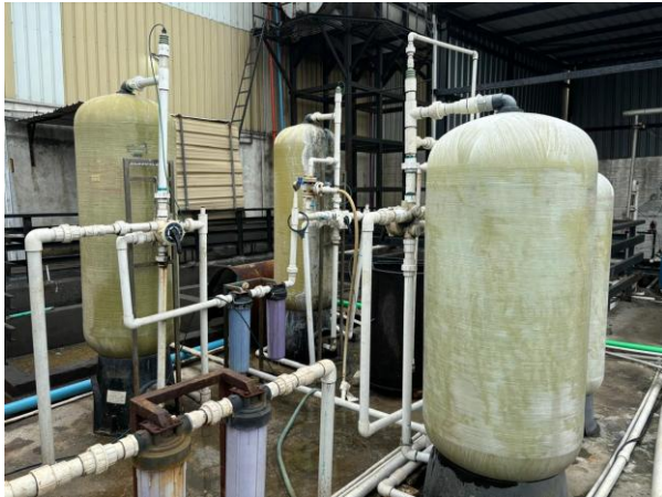
[Image 6; Filter Press (Sludge Water Extraction)]
