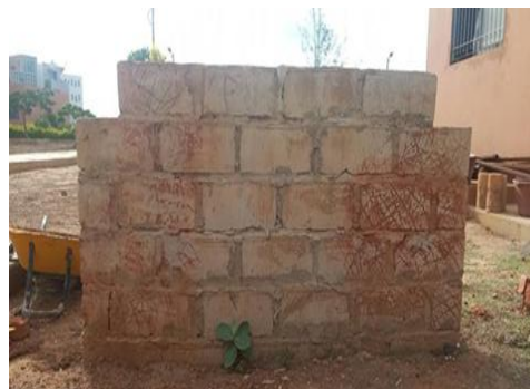
Figure 6: Cement support wall
