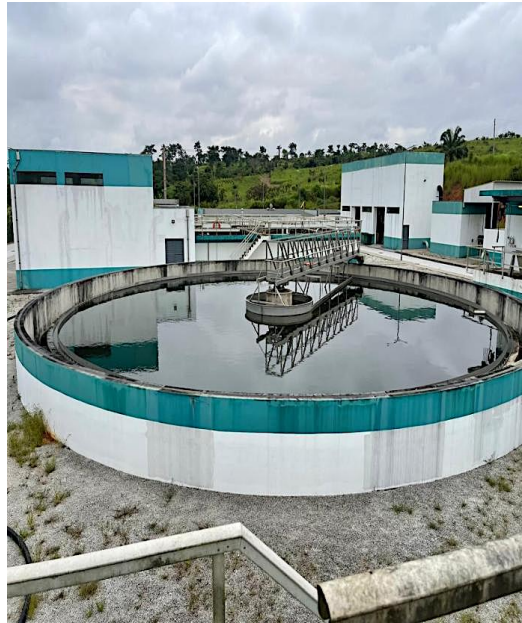
157 Figure6. Secondary clarifier of the Quilomosso WWTP.
