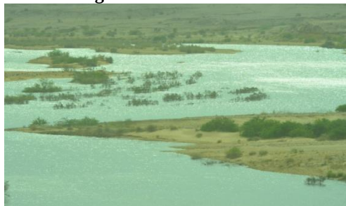
Fig. 1. A view of Darawat Dam
