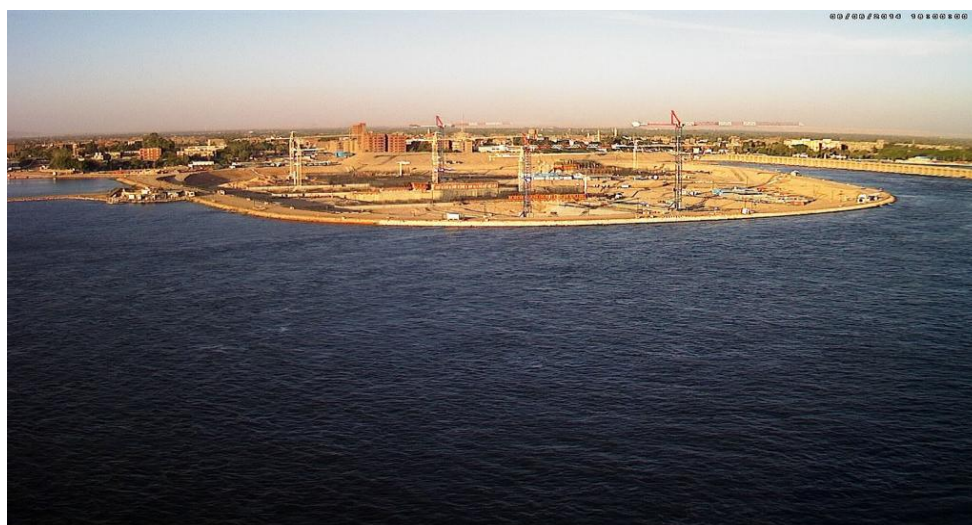
Figure (2): The construction pit for the New Assiut Barrage and Hydropower Plant
