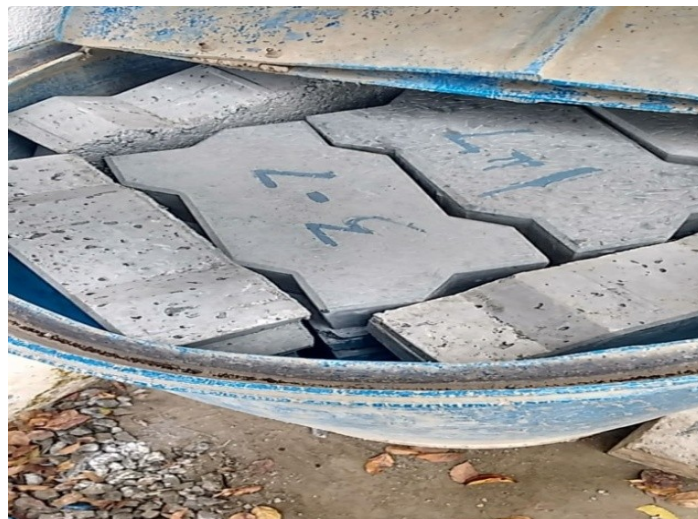
Fig III:- Curing of paving block.
