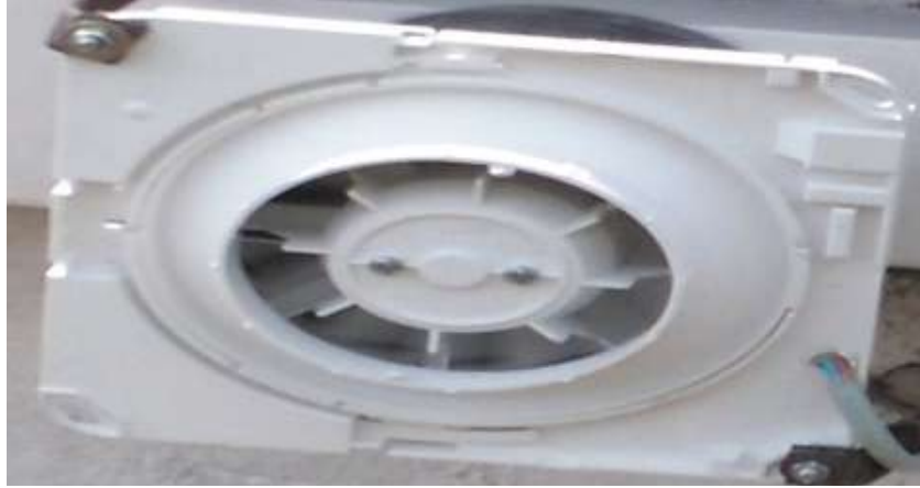
Figure 5:- Air extractor AP3102:80mm. 55m3/h. 23W.
