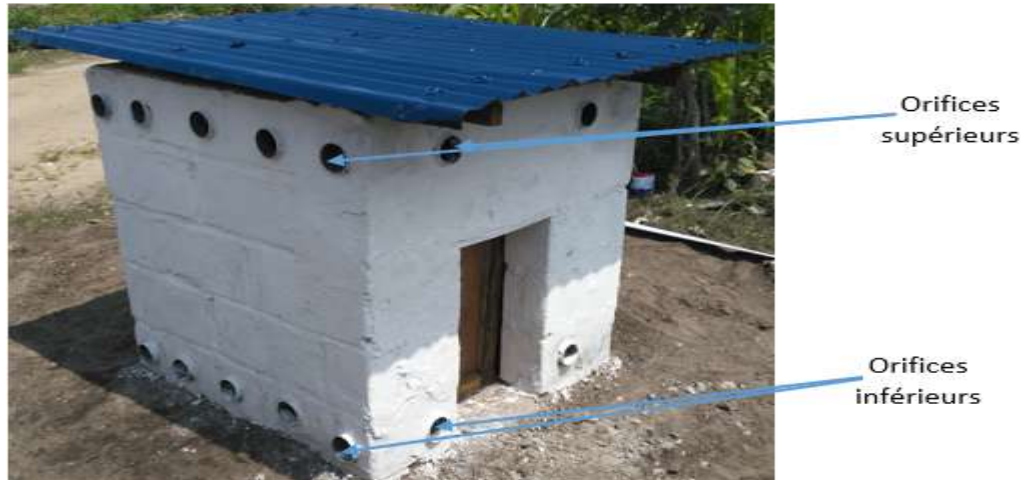
Figure 2:- Building built of perforated bricks and air circulation by natural convection
