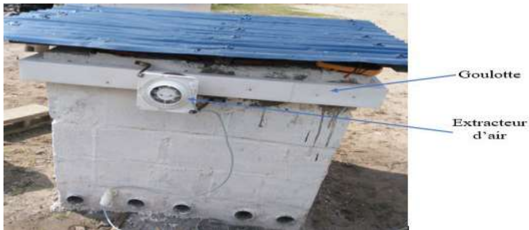
Figure 4:- A building made of perforated bricks equipped with a shaft with air extractor
