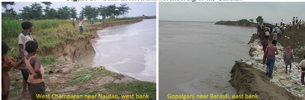
Figure 2:- Bank Erosion and Meandering of the Gandak.
