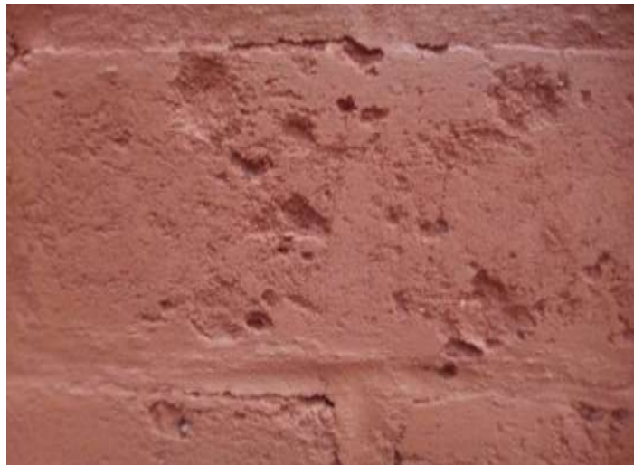
Fig. 13:- Quite marked effect of decrepitude of the wall (dosage of 5 and 6%).
