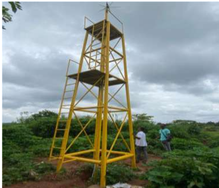
Figure 2:- The pictorial view of the installed wind turbine.
