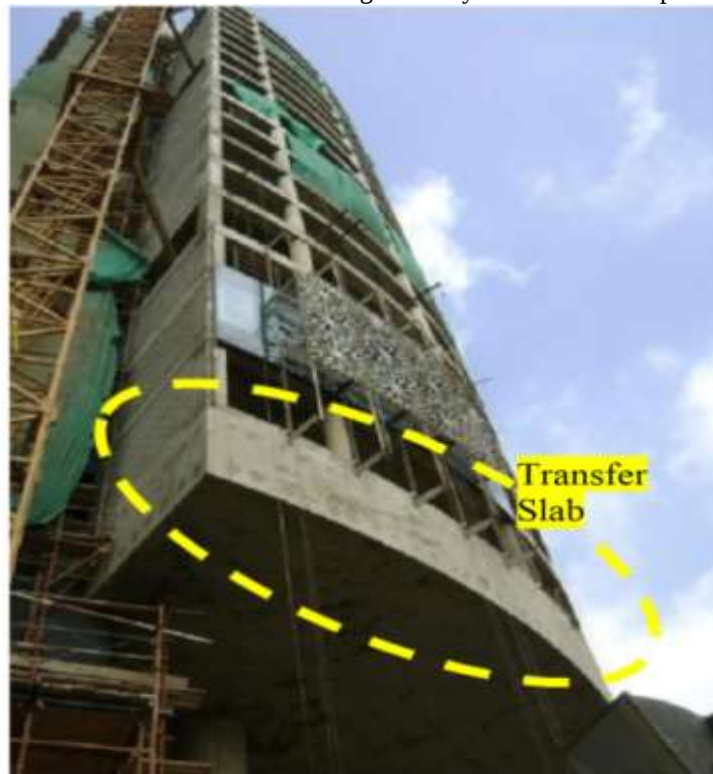
Fig. 1: High-rise building with a transfer slab.
