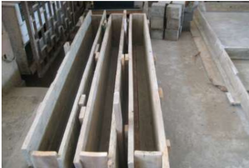
Fig. 3:- Wood Forms of Rectangular Beams.
