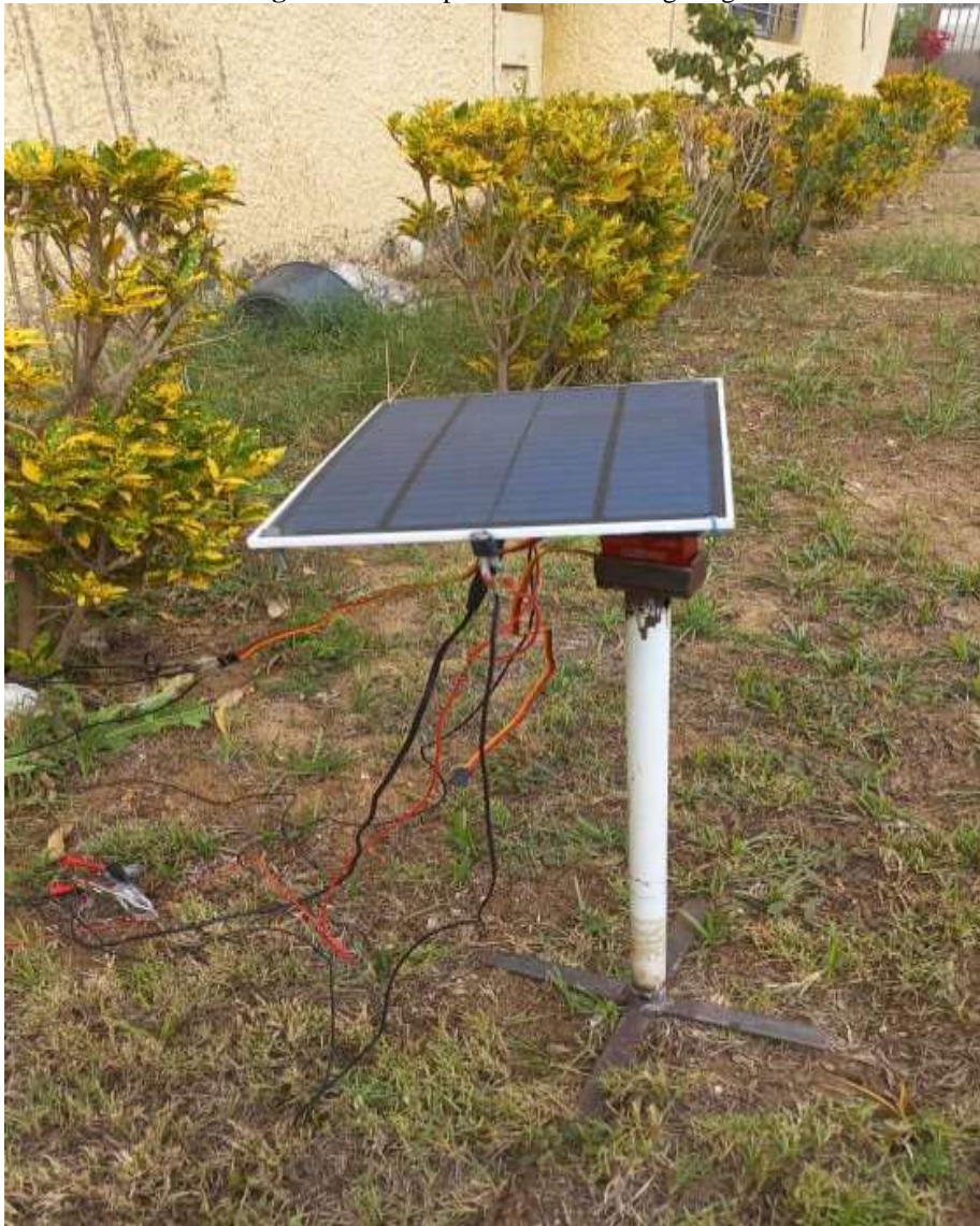
Figure 9:- Solar panel under solar lighting.
