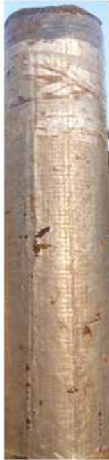
Figure 3:- Image of the tower chimney.
