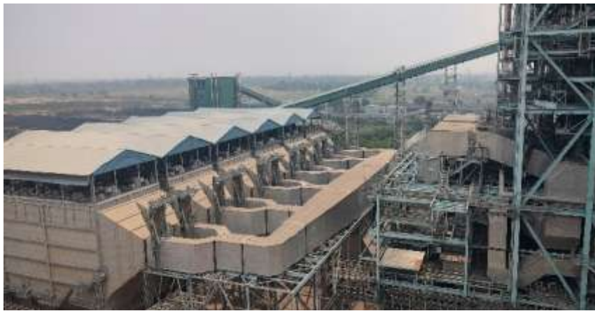
FIGURE 1.1 Boiler Duct Outer View
