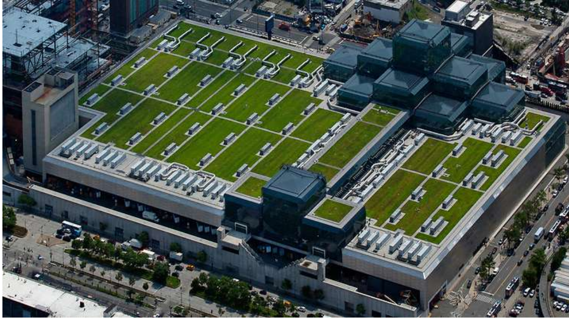
Figure 4:- Image of the Javits Convention Centre 7-acre green roof. Source: https://aerialarchives.photoshelter.com
