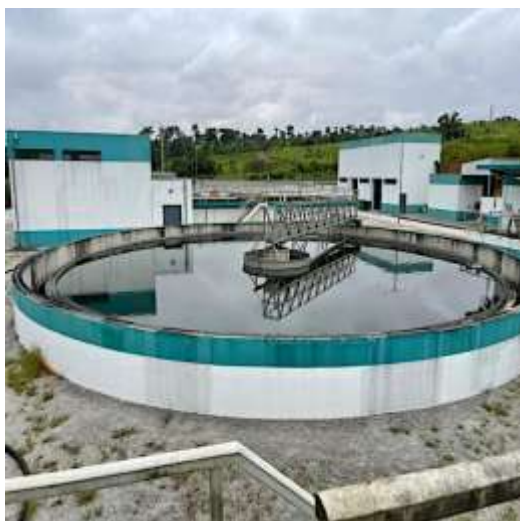
Figure 6. Secondary clarifier of the Quilomosso WWTP.
