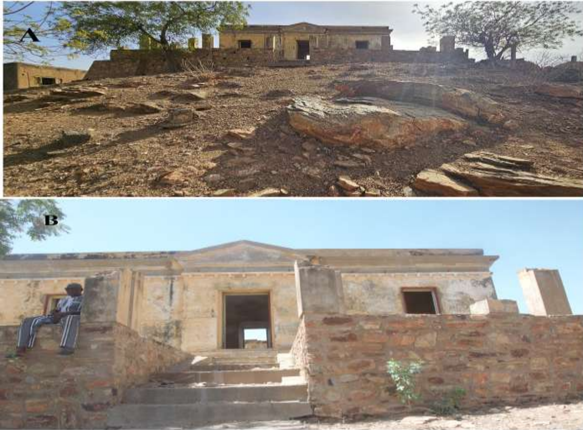
Fig. 4: Pavillon René Caillé. A: Building perched on a hill of sericite schist from the MBa1 formation; B: Detail of the main entrance.
