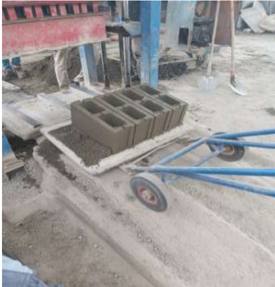
Figure 4.c: Removing the blocks from the moulds and moving them
