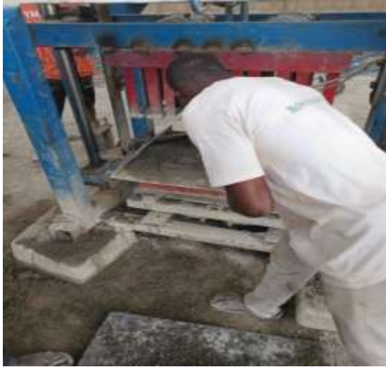
Figure 4.a: Pouring the mortar into the mould
