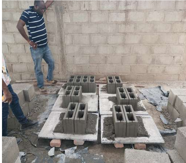
Figure 4.d: Storage of concrete blocks
