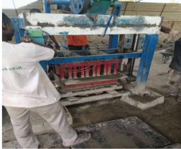
Figure 4.b: Compaction of mortar
