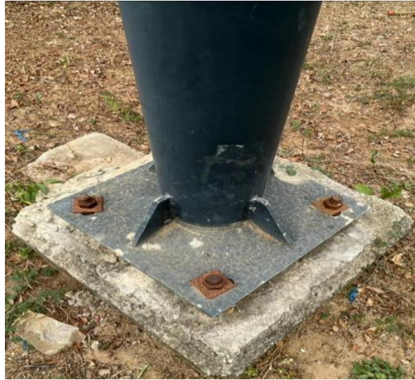
Figure 2: Streetlight pole base
