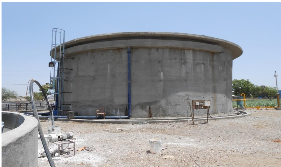
Photo No:01 UASB reactor at Prabhat Dairy, Shirampur
