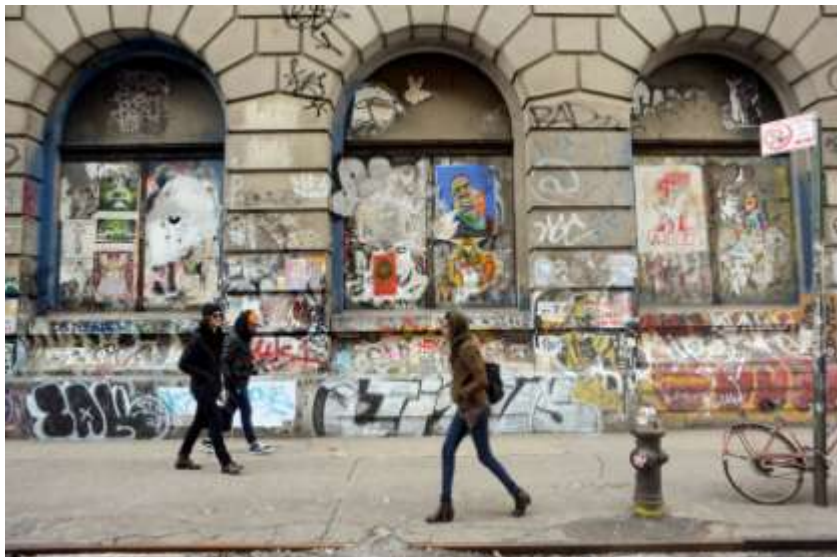
Figure2: An example of a building stained with graffiti. Photo: Casey Kellbaugh, New York Times.
