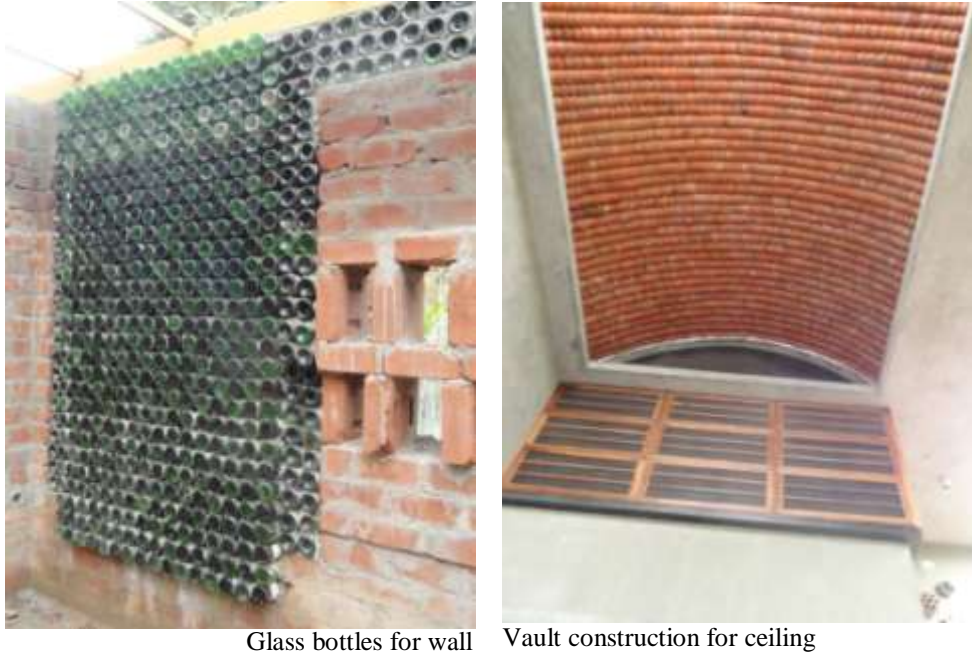
Glass bottles for wall Vault construction for ceiling
