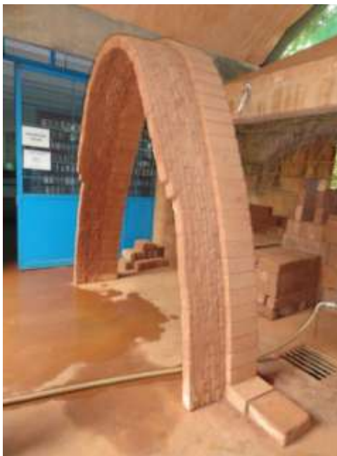
Brick horseshoe arch with corbelling
