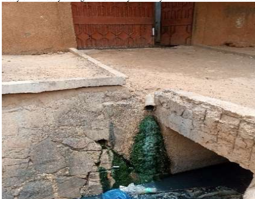
Figure 4:- Adjusting of the sinks collecting used waters of the showers of the households on the gutters (Source: Adamou Marafa M. (2021)).
