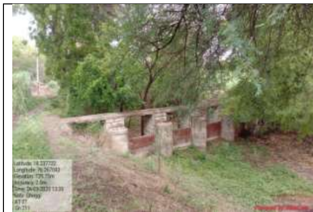
Existing K.T. weir, Village- Ghugi
