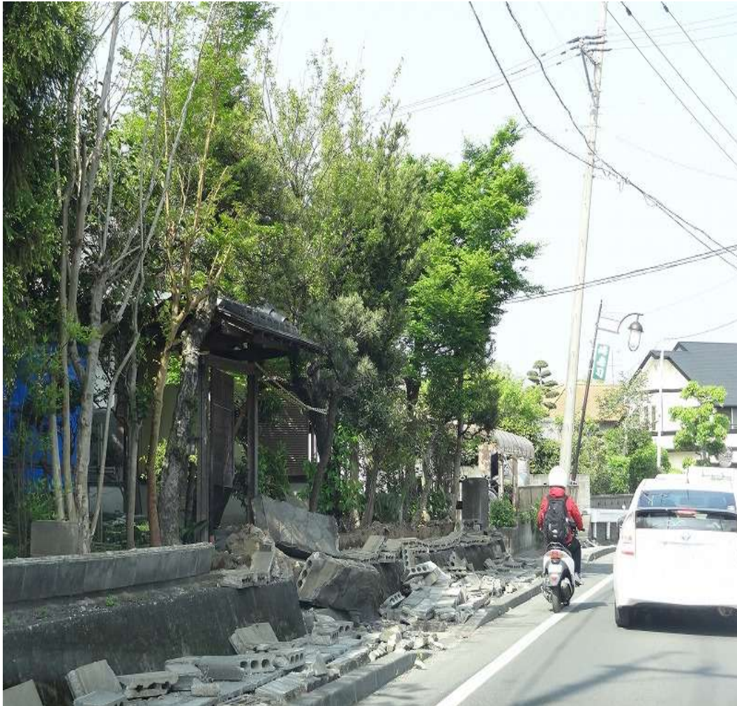
Fig 1:- Collapsed block wall on the sidewalk.
