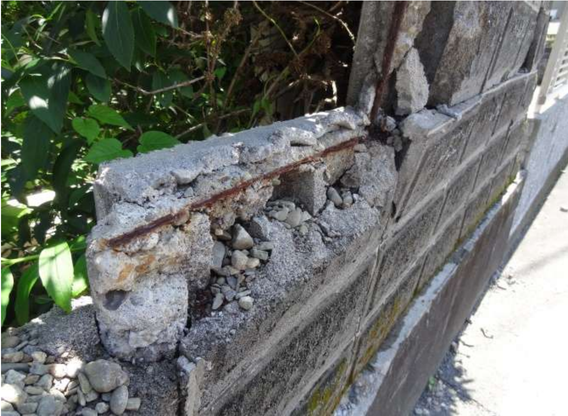
Fig 2:- Collapsed block wall with corroded rebars.
