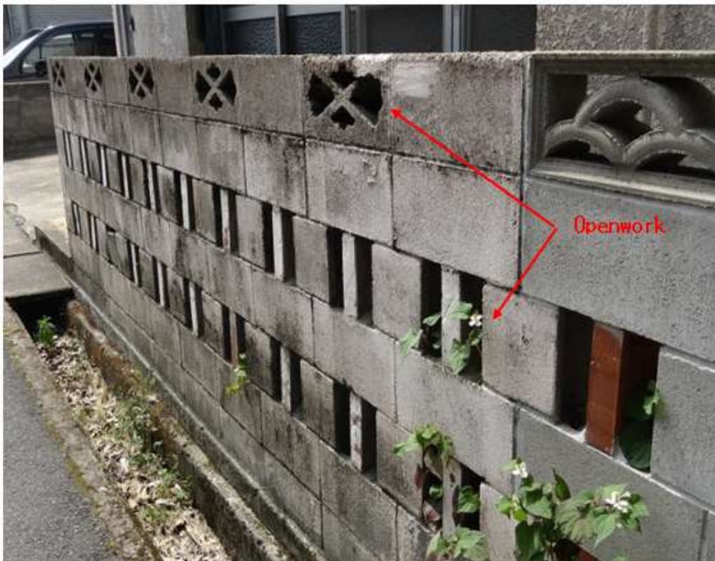
Fig7:- Block wall with openwork.
