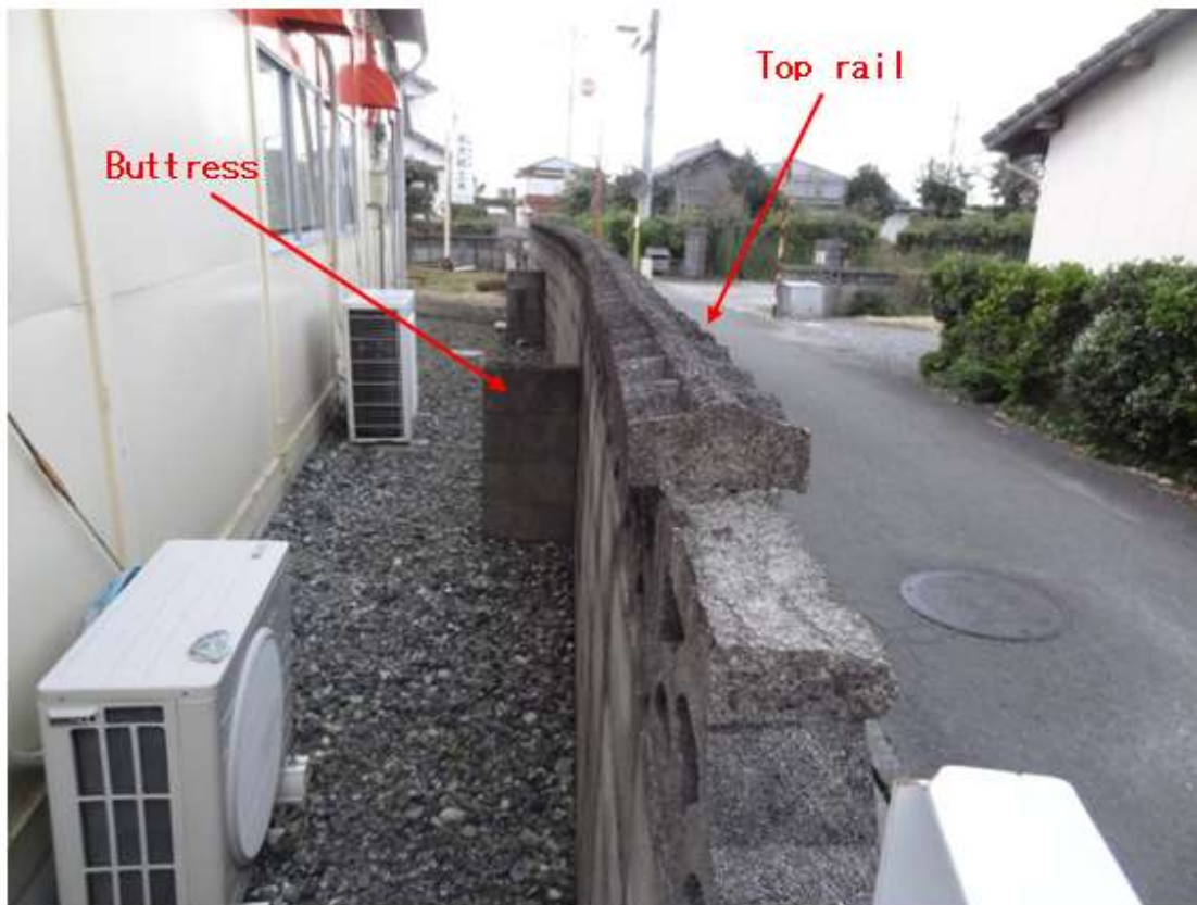
Fig 5:- Block wall with buttress and top rail.
