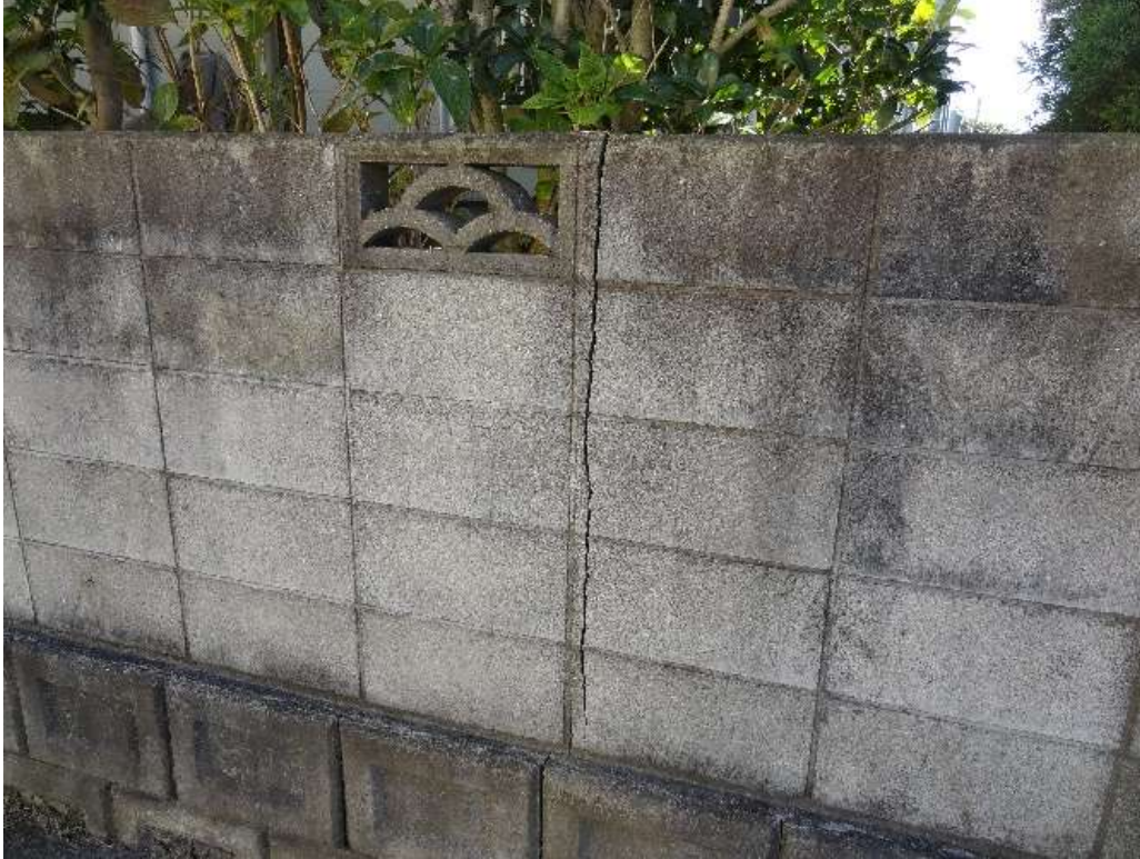
Fig 8:- Block wall with major cracks.
