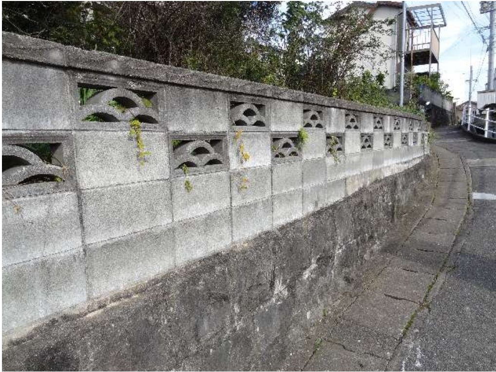
Fig 4:- Openwork block wall.
