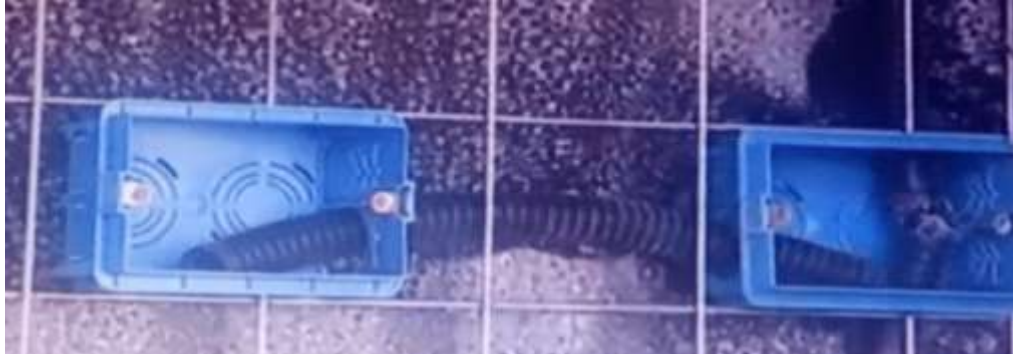
Figure 12:- Installation of electrical conduits.
