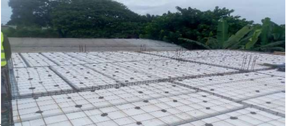
Figure 14:- Floors awaiting concreting.
