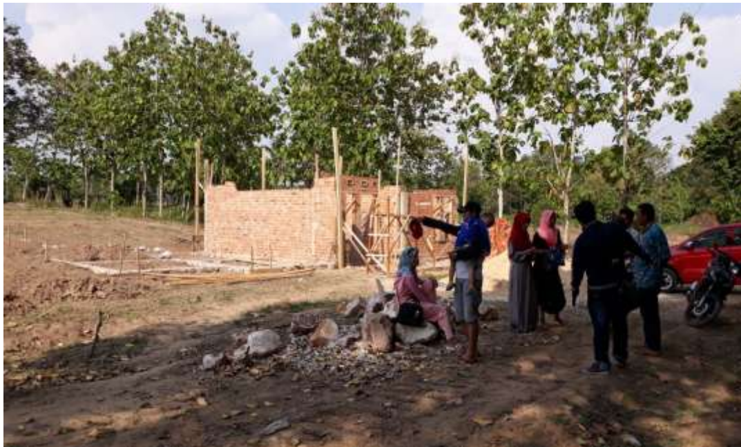
Figure 1:- Initial Housing Location, Limited Construction, Only a Sample House Available.
