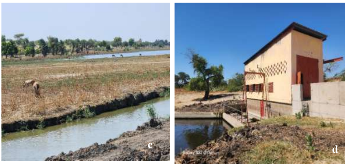
Figure 12:- Various Methods of Soil Salinity Management in Reclaimed Polders (a) Leveling with small dikes for irrigation in this wheat plot, (b) salt precipitation on the surface, (c) drain surface (d) utilization of a pumping station.
